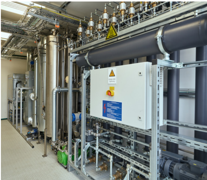
The system can be switched to an electrolysis mode, which allows electrical energy to be used to produce hydrogen and methane.
