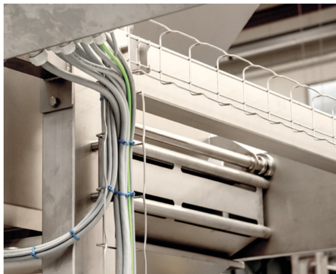
Screened cables that prevent EMC disruptions between the individual plant parts are often needed.
