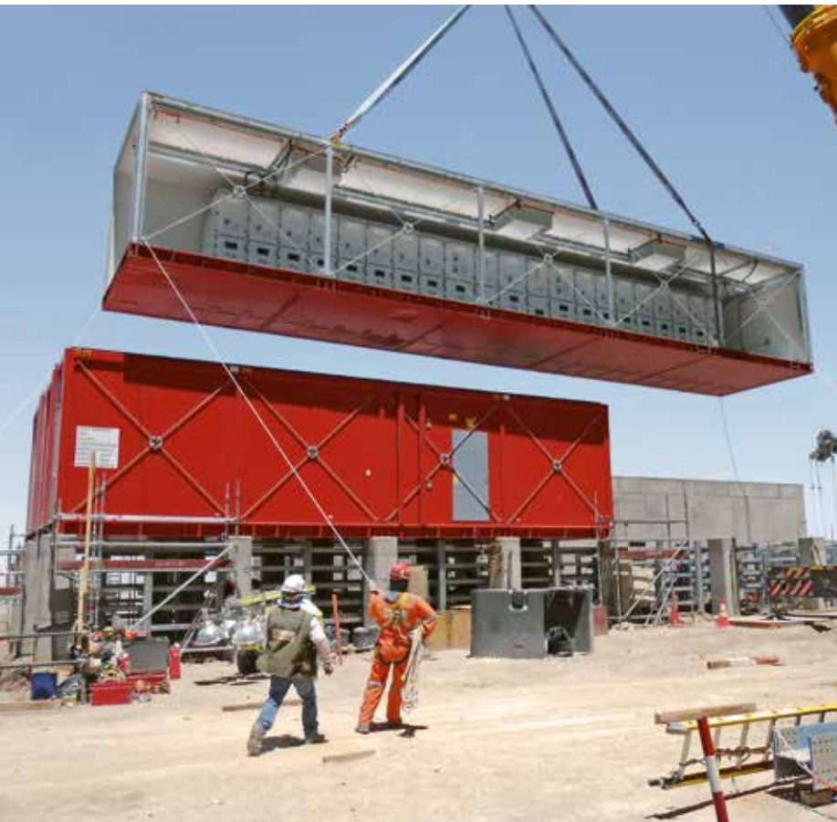
Containers are often connected to form plant structures.
